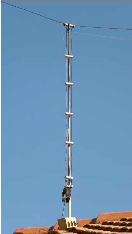
11 m Band "Zepp" (EDZ) antenna: 450 ohm Ladder Line
